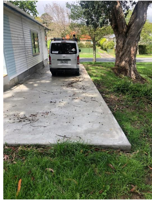
Photographs 1 and 2. Car-parking pad recently constructed within the root zone of four of the Eucalyptus trees.
